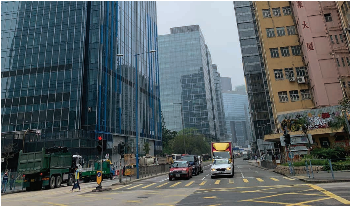
New GradeAoffice vs Old insutrial buildings
